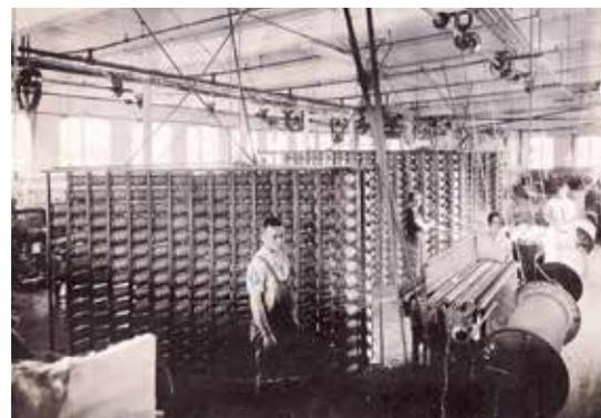
The Weave Room, shown in 1930, had one big electric motor in the ceiling powering a long shaft, from which various leather belts would transfer that power to each successive machine in the room.
