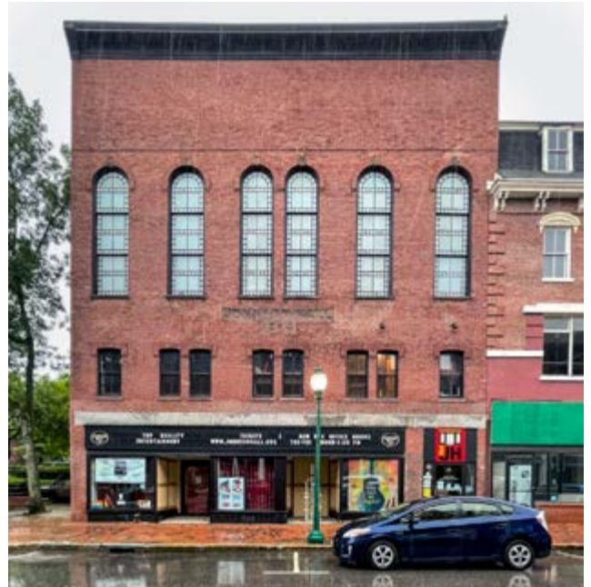
April marks the start of extensive renovations to the Johnson Hall Performing Arts Center at 280 Water St. in downtown Gardiner, photographed above in July 2021. The iconic facility is expected to be closed for at least 18 months.
