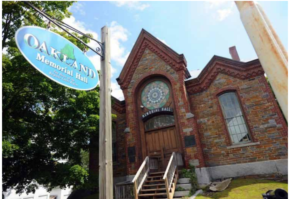
A renovation project expected to cost as much as $5 million is intended to breathe new life into historic Memorial Hall in Oakland, a 1870s structure, which is one of four Civil War memorial buildings in Maine.
