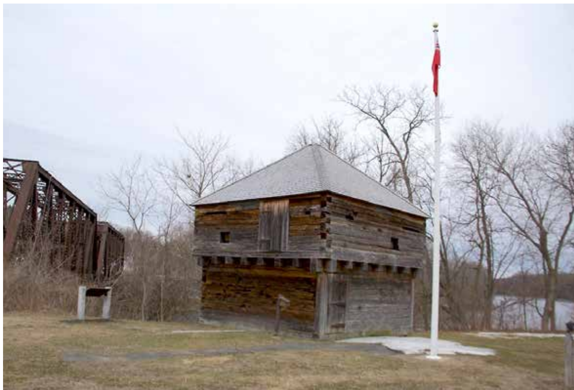
Fort Halifax's reconstructed blockhouse stands on the north bank of the Sebasticook River in Winslow.
