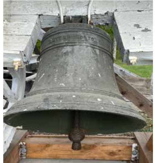
The Benton Falls Meeting House's Revere bell rests on the ground next to the building, awaiting the restoration of its decaying belfry.
