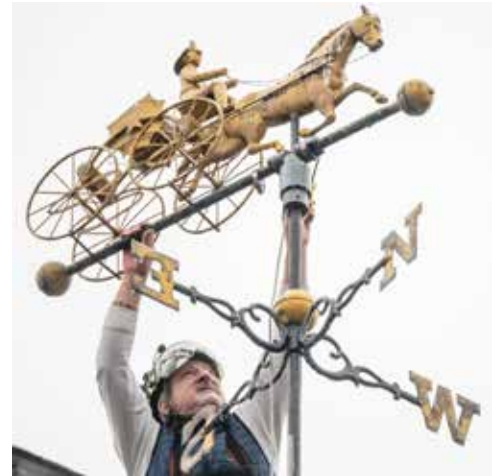
Harry Wolfington, owner of Pinnacle Tree Professional Arborists, works to remove a weather vane April 6 from a Hallowell building that used to house the fire station on Second Street. He ended up cutting the post underneath it to get it down
