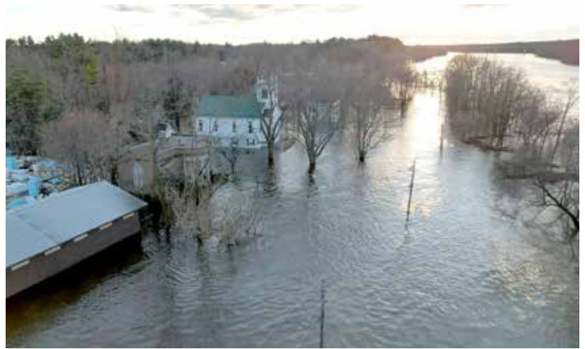
Floodwater from the swollen Kennebec River surrounds buildings in late December on Lithgow Street in Winslow. The Taconnett Falls Genealogical Library's brick building, partly screened by trees in this aerial photo, can be seen just below the Winslow Congregational Church.
