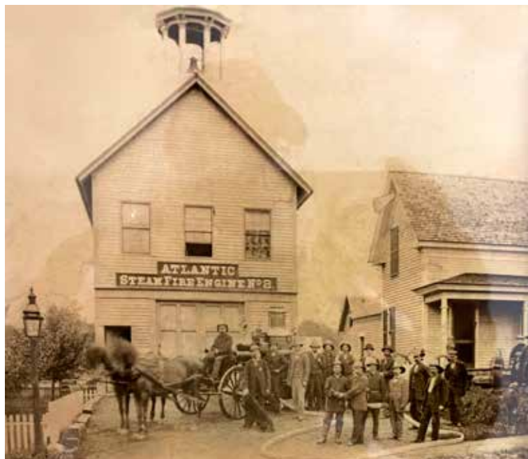
The Cony Street fire station, shown here in its early years, had a round cupola and an open-gable roof when it was built. During a later renovation, the cupola was removed and the roof was made flat.
